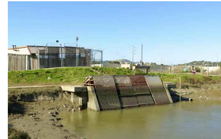
Existing tide gate and pump station at Shorebird Marsh. A tide gate across San Clemente Creek would likely look different.
